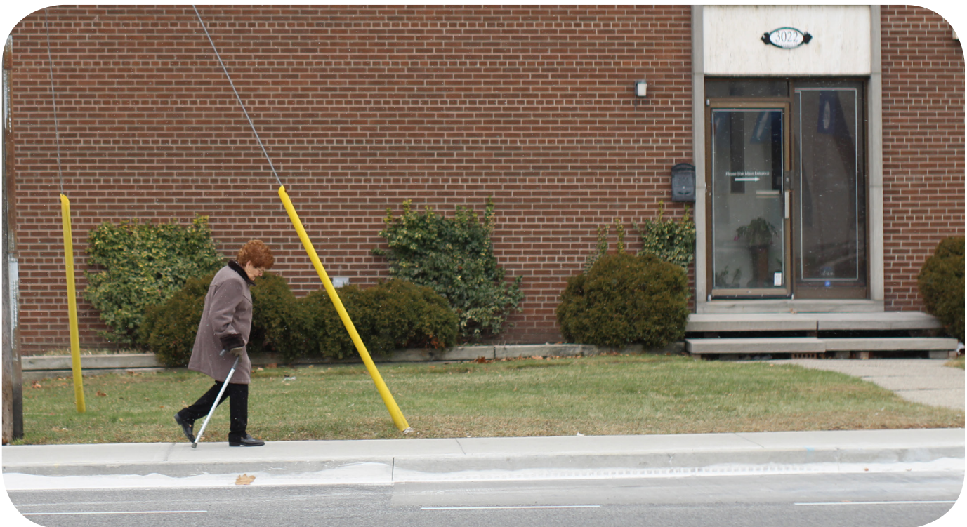
Figure 9. Some barriers are hidden in plain sight. Stairs without railings make the entrance inaccessible.
